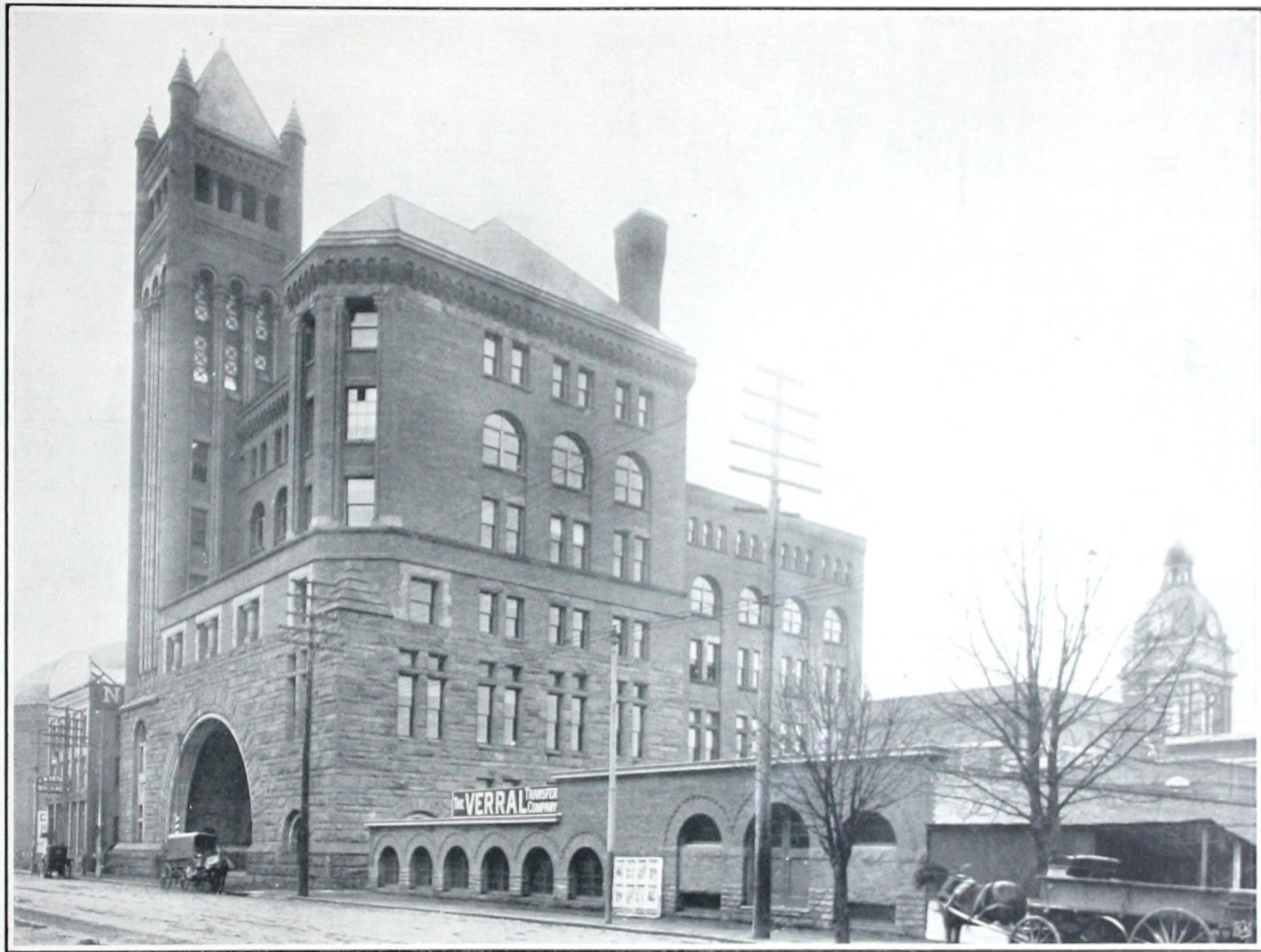
Fig. 191.—Union Station, Toronto In which the "Hayes" Patent Lathing was used.
